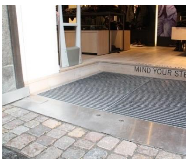
Level floor, ready to enter/exit
