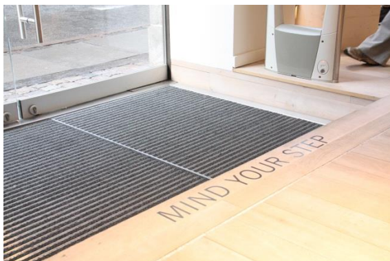
The HDN lift ready for operation at the lower level
